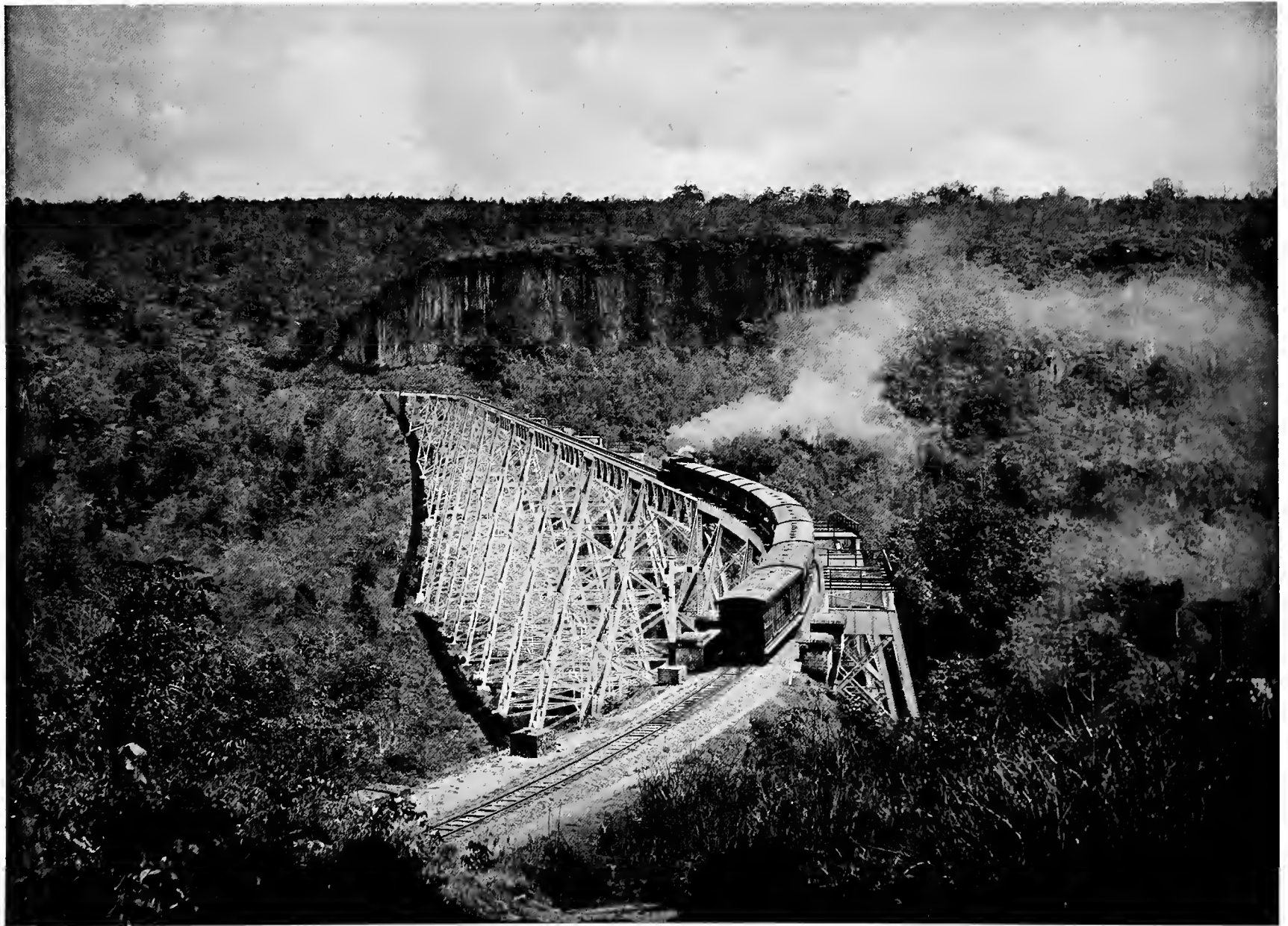
The Gokteik Gorge and Railway Bridge
